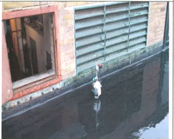
Roof sample location.
